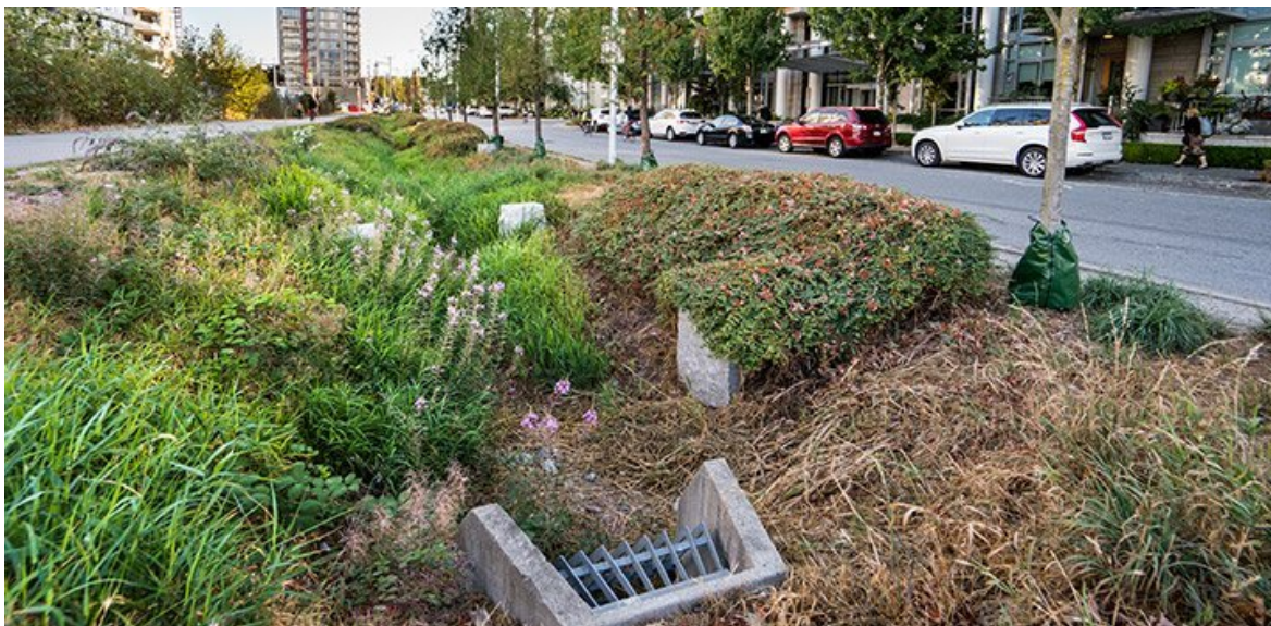
Figure 4. Diagram of a swale, which uses native plants and grasses to decrease flooding and erosion, stimulate proper drainage, and mimic a natural wetland to filter rainwater and runoff. 40
